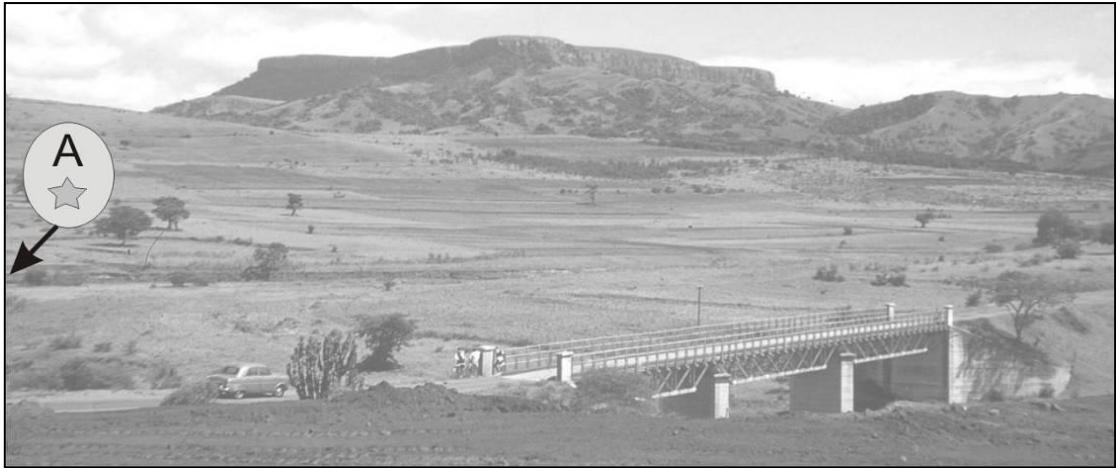
Above: Dusi Bridge as it appeared in the 1950s, with very little habitation. The pump station had not yet been constructed.
